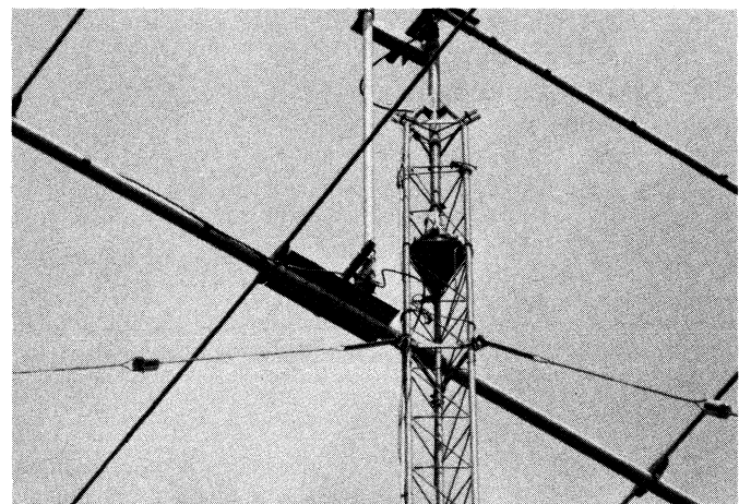
The guy-wire torsion bracket is mounted just above the bottom rung of the tower top section. The 10-meter antenna rotates just above the top set of guys. An empty torsion assembly at the top of the tower is available for an additional set of guy cables if they should be necessary.
